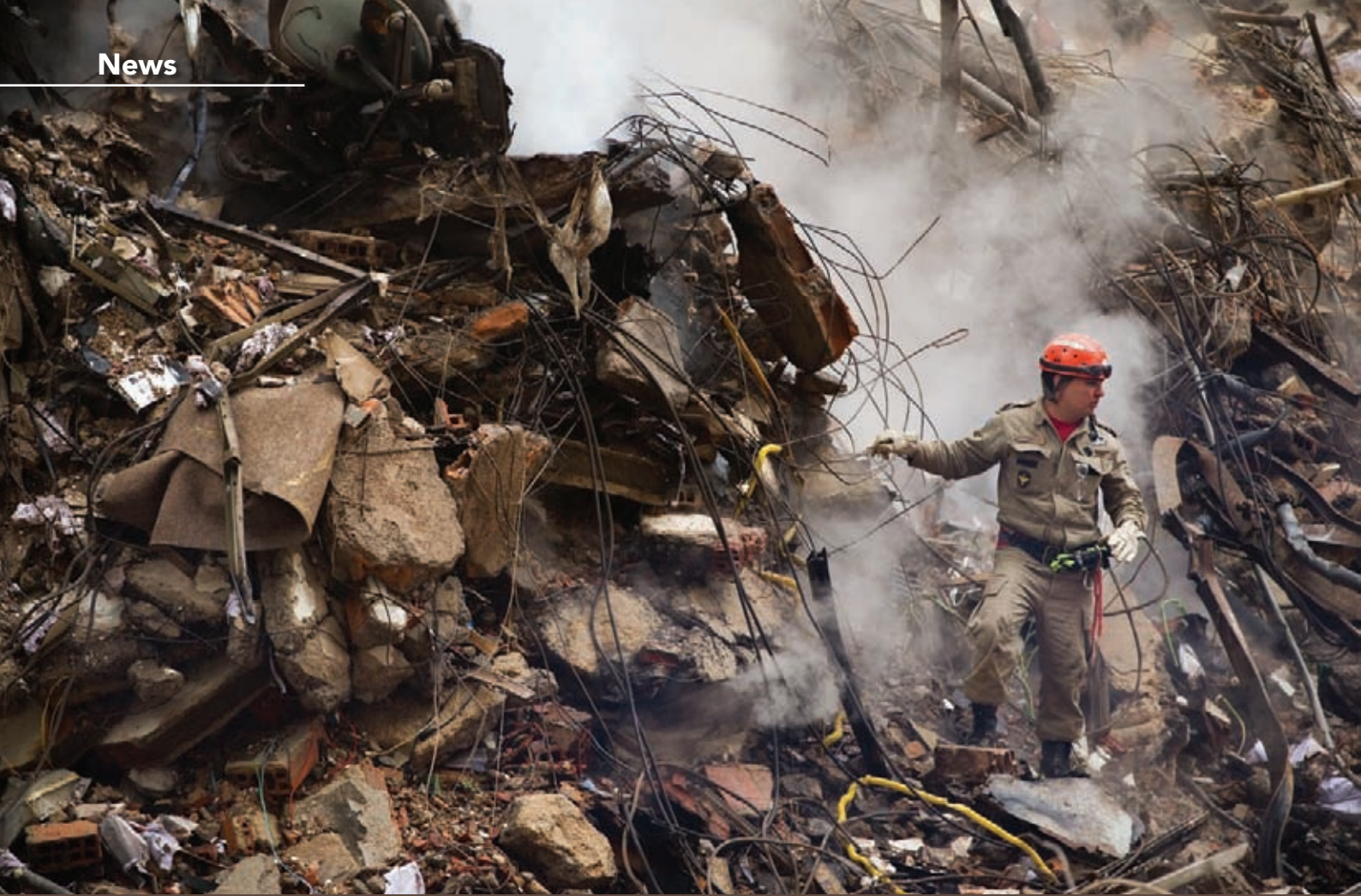
A fire fighter stands in the rubble of a building that collapsed in downtown Rio de Janeiro, Brazil
