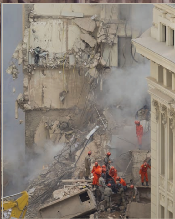
17 people were killed in the building collapse
